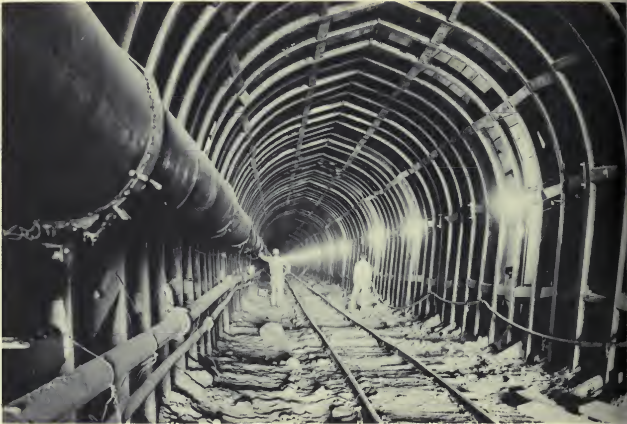
MAN-MADE CAVERN is the Frenchman Hills tunnel, 16 feet in diameter, shown above. Puddle of water inside tunnel, at left, is hardly a forerunner of things to come, when enough water to irrigate 50,000 acres will pour through the structure. All photos by Harold E. Foss, Region 1.
